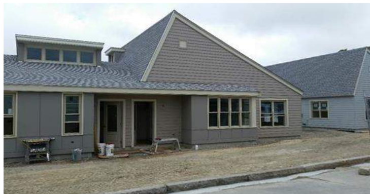
WESTWOOD - Above, Westwood “Before” (30 1-BR “Barracks-Style” Units). Below, Westwood “After” (12 Accessible 705-Family Units)
