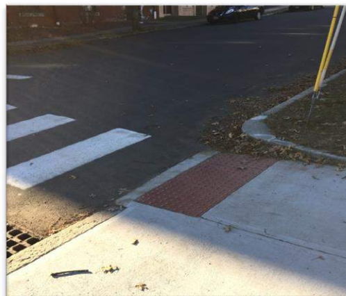
The town of Montague received a $35,000 Municipal ADA grant to improve failing sidewalks. At right, the improved, accessible intersection, including new tactile paving.
