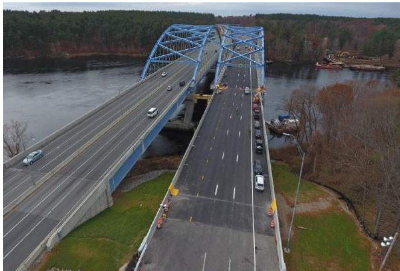
The Whittier Bridge/I-95 Improvement project replaced the existing bridge and widened and improved a 4-mile section of I-95 in Newburyport, Amesbury, and Salisbury, while replacing four adjacent bridges. The project was completed in 2018.
