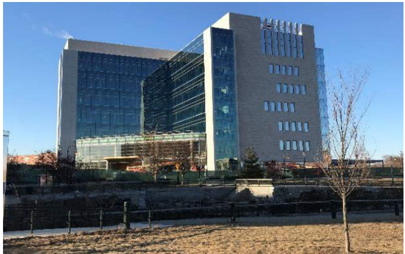
Construction of the new Lowell Justice Center, designed for high energy efficiency and funded in DCAMM’s capital plan, is nearing completion.
